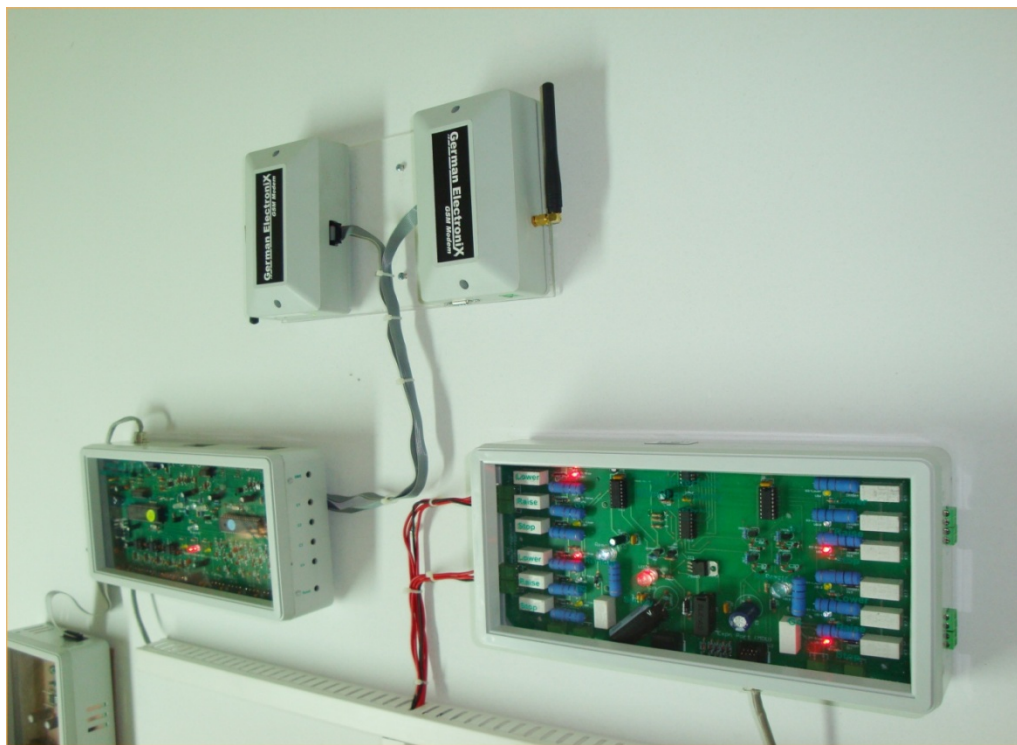
FIGURE 1 MDU UNIT, GSM MODEMS, PUMP INTERFACE, POWER SUPPLY SOLAR CONTROLLER
